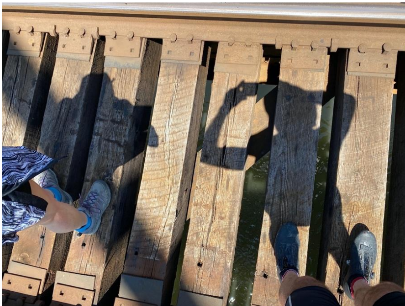
Railroad Bridge over the Genesee River between Orleans and Canandaigua, NY.
